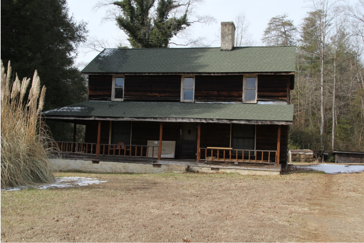
Rhoney-Sain House, facade, view to west
