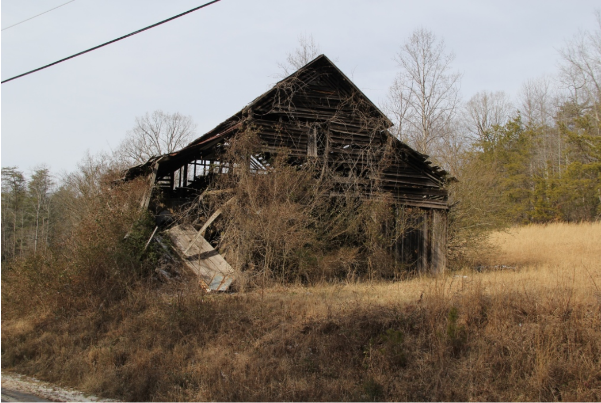
Barn, east elevation, view to northwest from Rhoney Road
