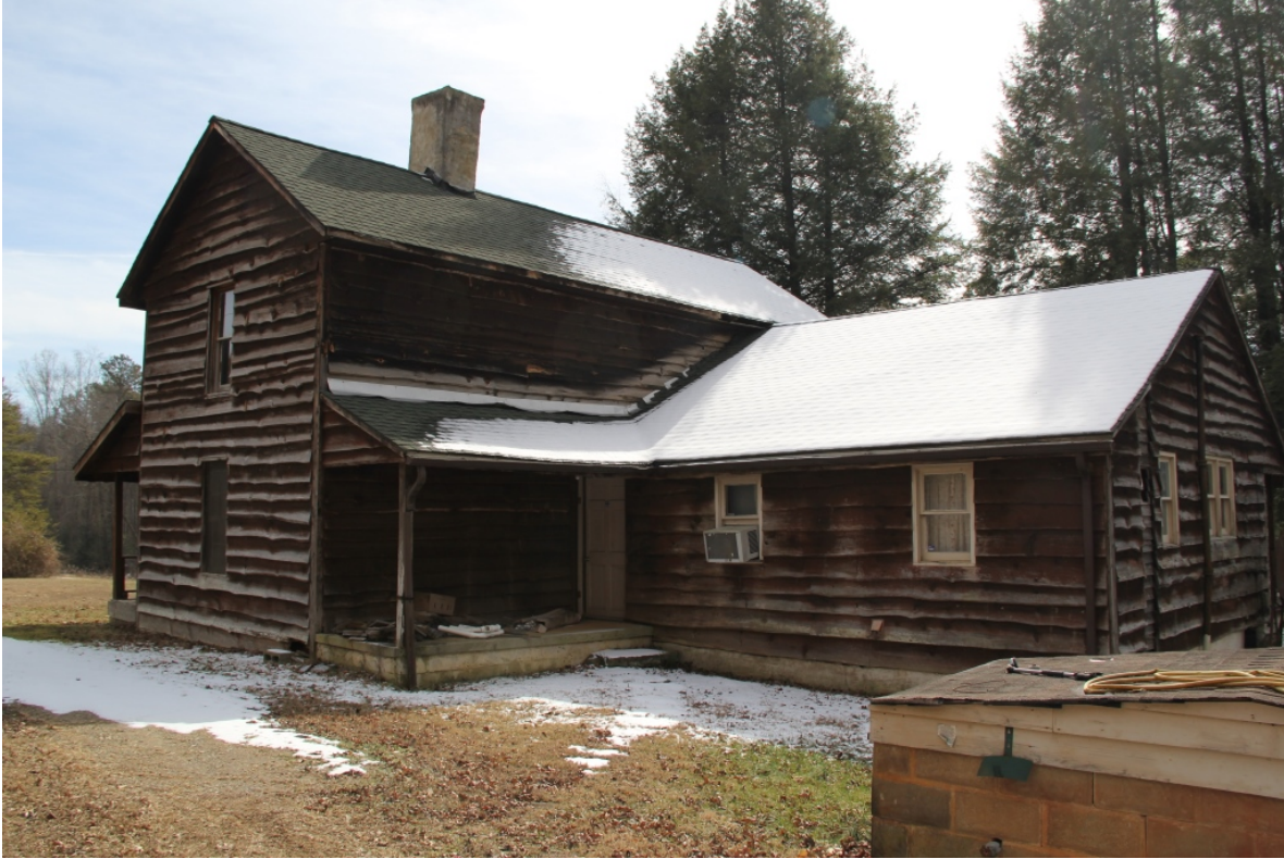
Rhoney-Sain House, oblique rear view to southeast
