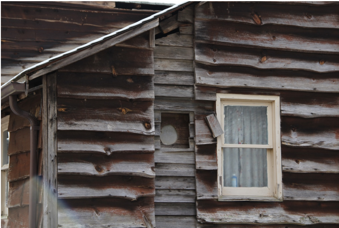
Rhoney-Sain House, siding detail, west elevation of rear ell
