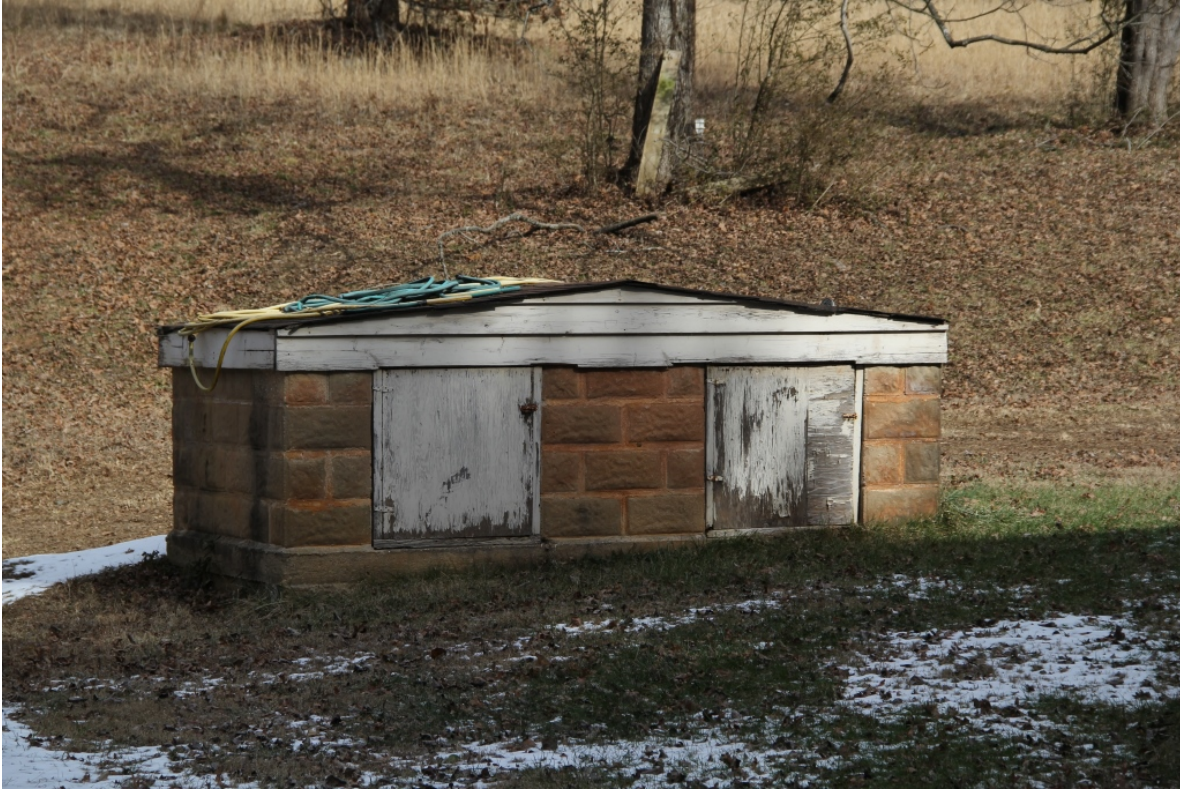
Well house, south elevation, view to north
