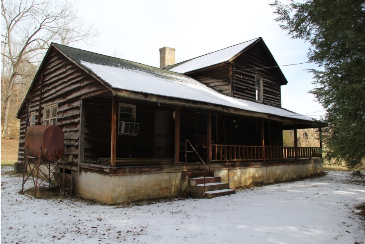
Rhoney-Sain House, oblique rear view to northeast
