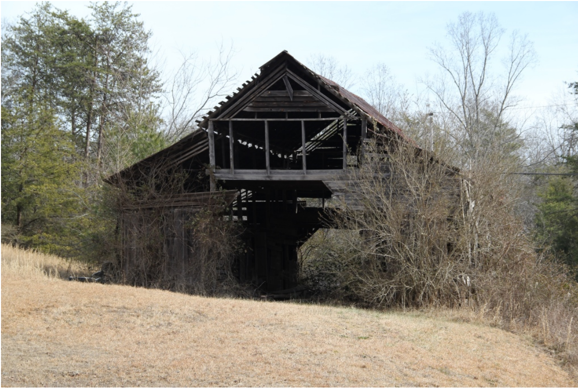
Barn, west elevation, view to east
