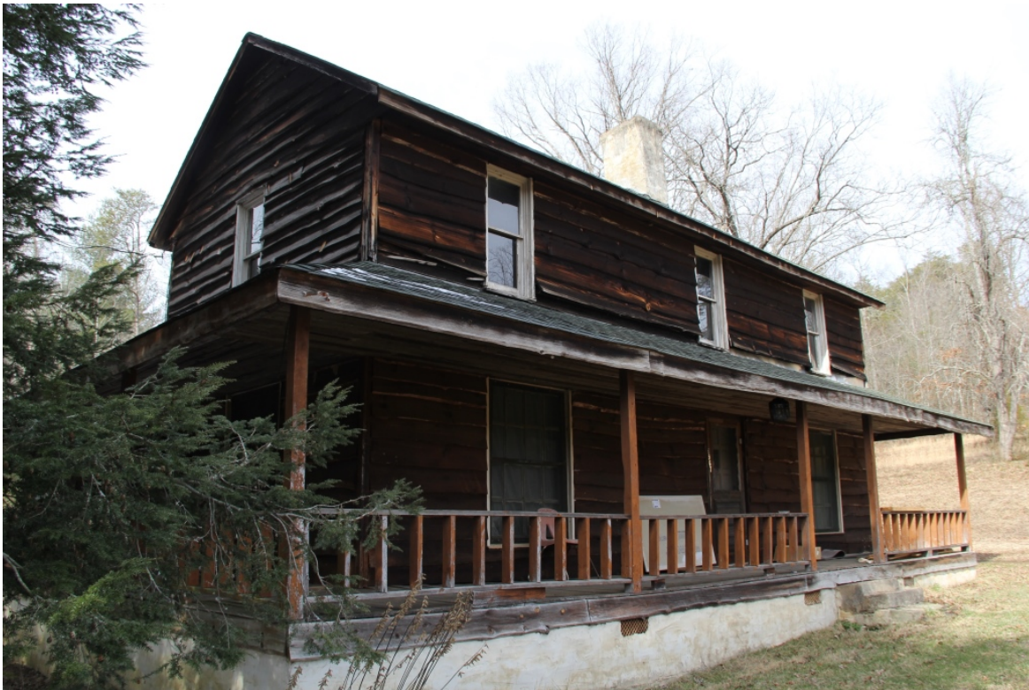
Rhoney-Sain House, oblique front view to northwest
