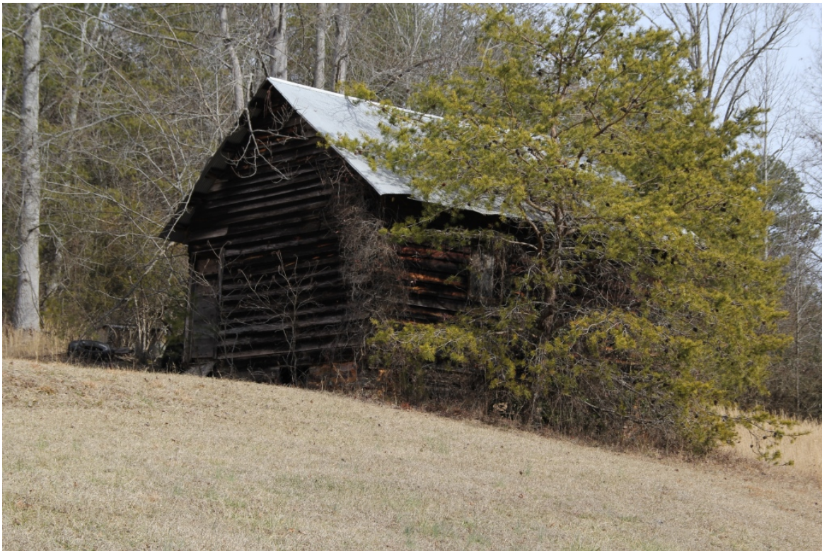
Crib, oblique front view to northeast
